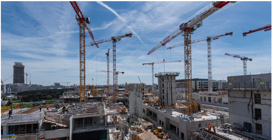
Construction site of the Olympic and Paralympic Village
